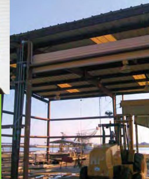
In this case, the building was designed as an enclosed structure. Contrary to popular belief, you should close all doors and windows prior to a storm. It is a common misconception that allowing air to flow through doors or windows left partially open will reduce the pressure or force on the structure.
