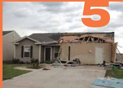
“... and the total removal of the garage. This now leaves the attic as an opening to create internal pressure and continue the process. In essence the building is deconstructed by the tornado.”
