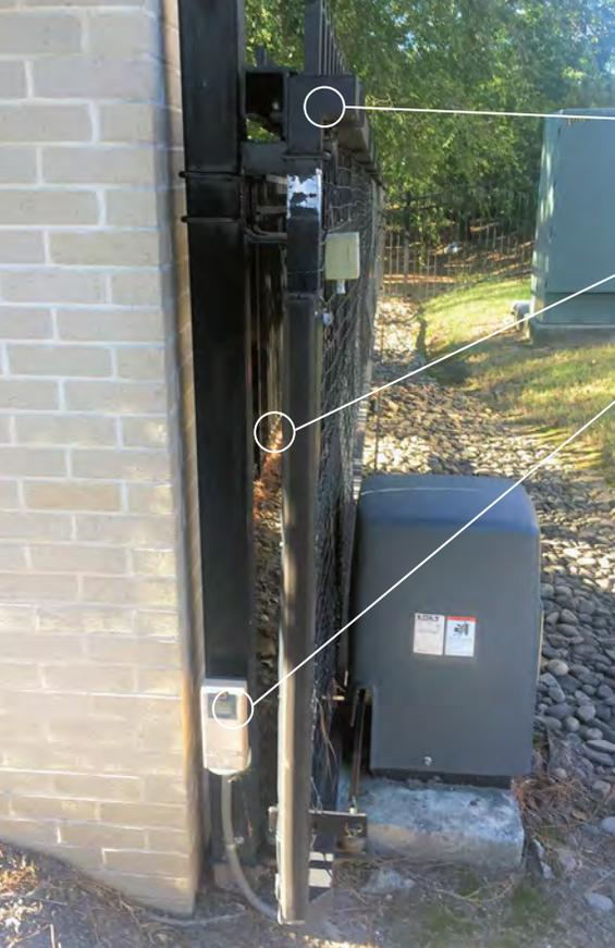
7. No exposed weight-bearing rollers
