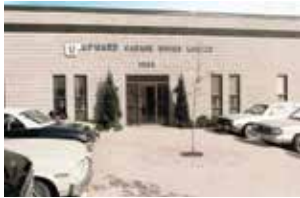
First building, ca. 1980.
