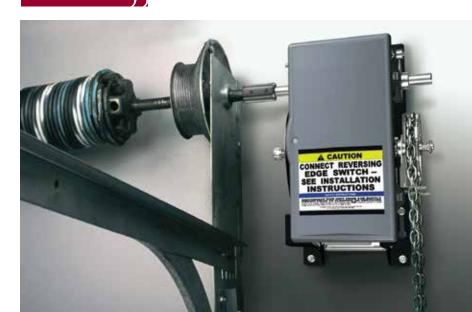
Jackshaft operators can be connected to any door that has a shaft as the driving element. That includes rolling doors, rolling grilles, high-speed fabric doors, or multi-leaf doors.
