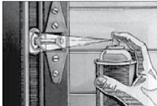
**Lubrication** Regularly lubricate the moving parts of the door. However, do not lubricate plastic idler bearings. Consult the door owner's manual for the manufacturer's recommendation.
