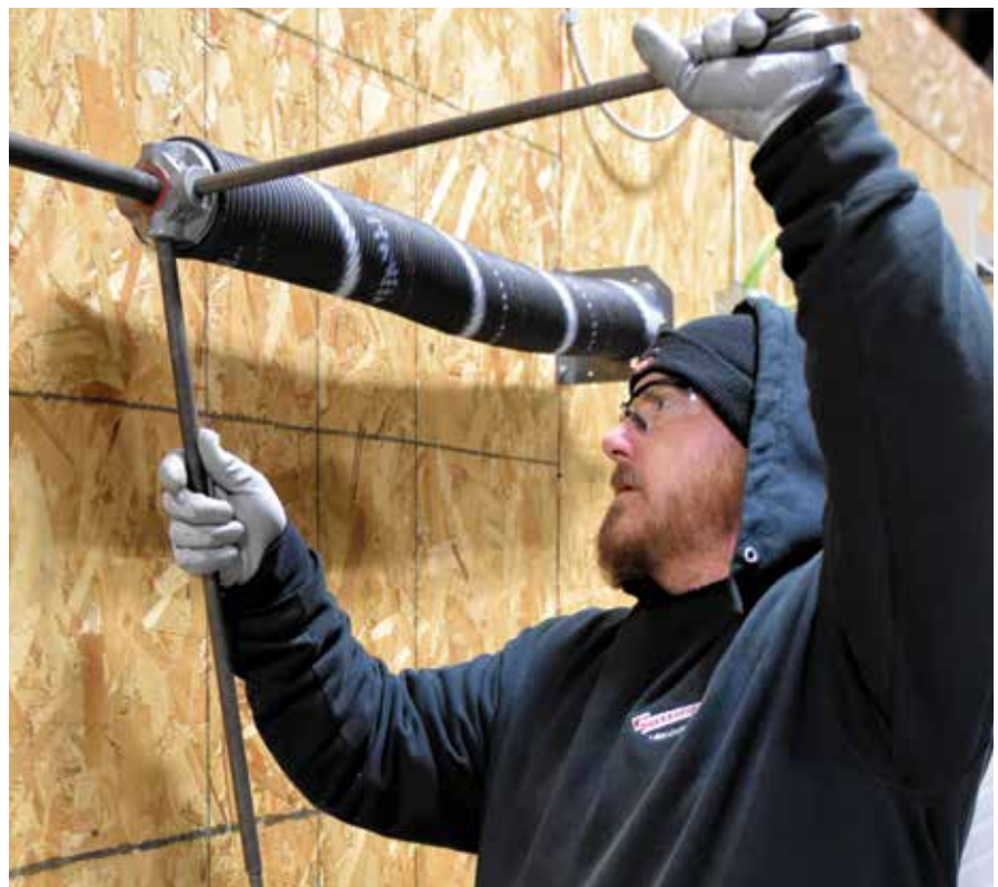
WINDING RIGHT: When using winding bars, grip the bar with your palm facing out and away from your head, not with your palm facing in. Pictured: Dustin Stone.
