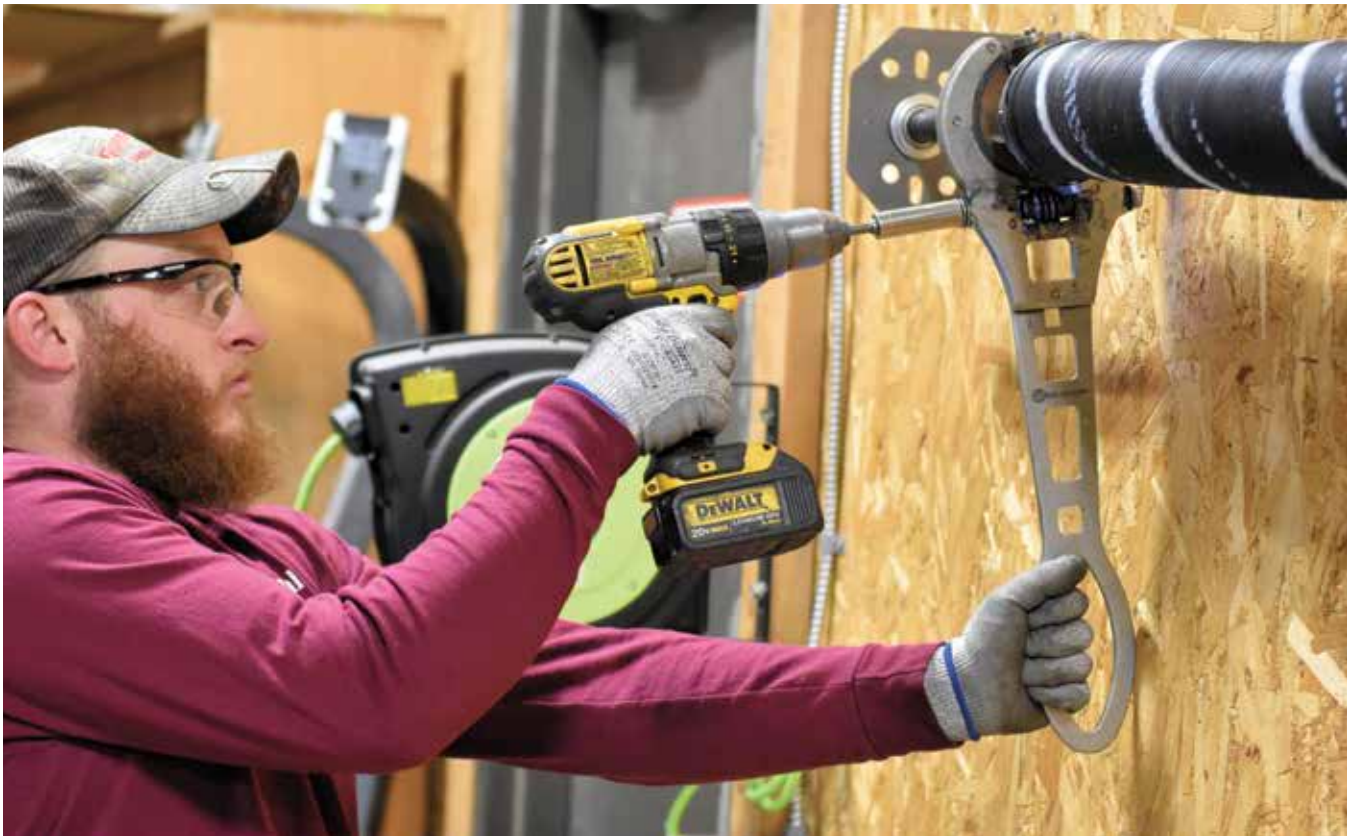
WINDING BY DRILL: Tyler Firestone demonstrates how to wind springs with the Surewinder and a drill.
