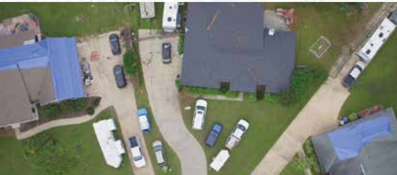
After Hurricane Sally (2020), this home with a Fortified Roof suffered no damage while neighbors on each side needed extensive repairs.
