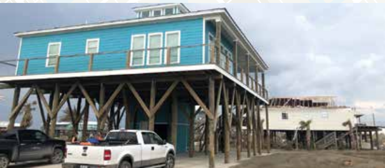
Owners of this Fortified Gold home on Grand Isle, L.A., were able to return home the day after Hurricane Ian (2022) destroyed hundreds of homes in the community.
