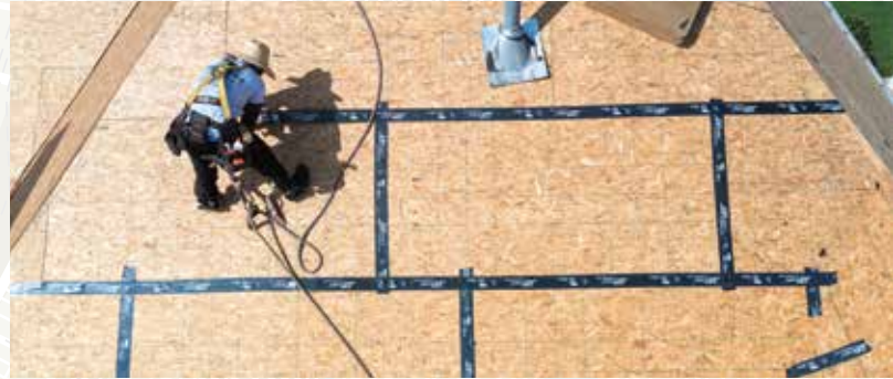
Sealing the roof deck is a key requirement for Fortified Roof and can reduce water intrusion by as much as 95%.
