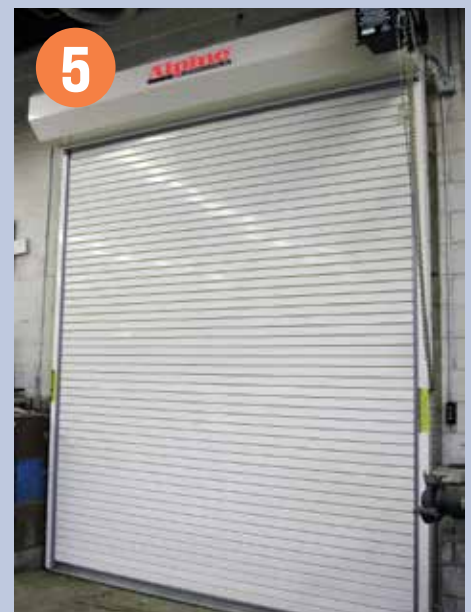
This door is powder coated which helps protect against scratches, corrosion and fading
