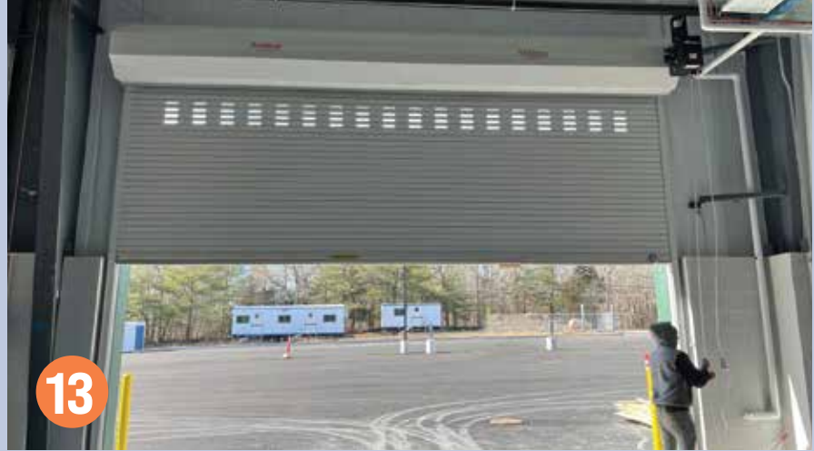
A technician tests the hand chain after the installation has been completed.
